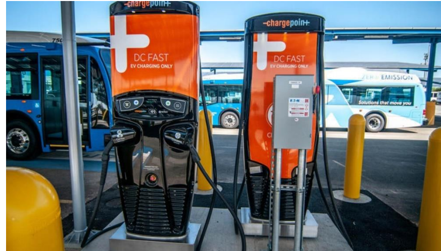
Exhibit C.1.6 Depot-based DC fast chargers (Level 3)
